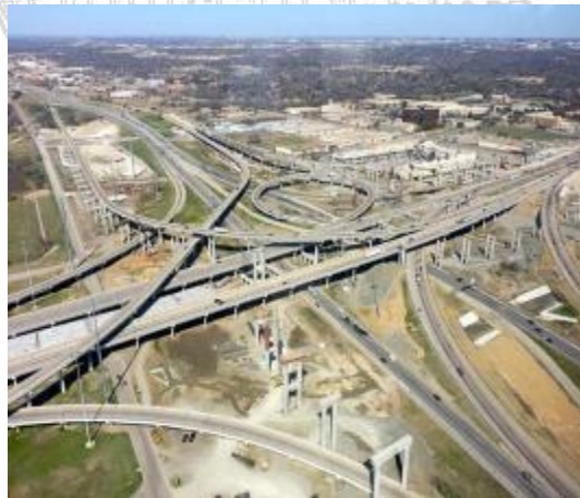
IH-635 Managed Lanes (New LBJ) Dallas, TX
