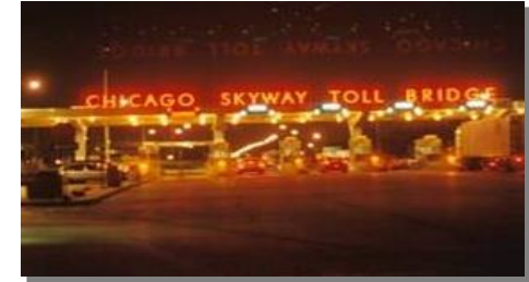
Chicago Skyway Toll Bridge Chicago, IL
